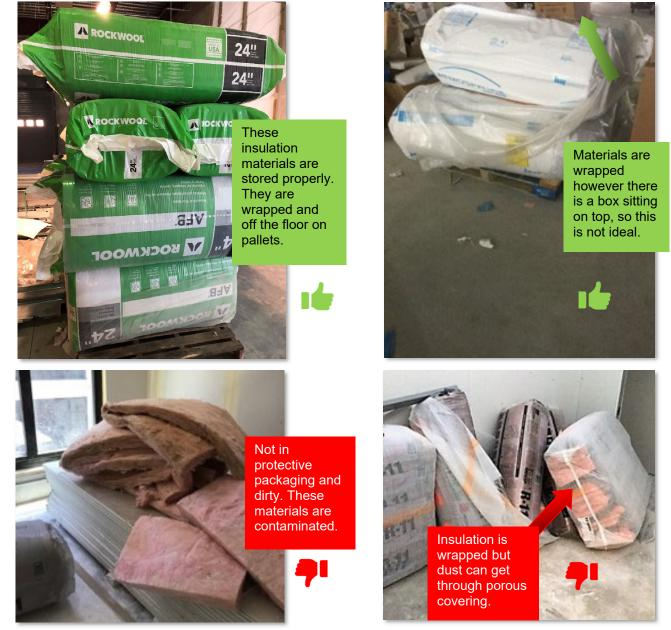
Absorptive building materials such as porous insulation, wood, gypsum wallboard, should be kept dry to prevent the growth of mold and bacteria. Cover these materials to prevent water damage, contamination from dirt/debris, and store raised from the ground. Do not stack other materials on top. During installation, minimize the time material is in contact with floor or other porous materials. Immediately remove materials that show signs of mold and mildew or moisture stains.
